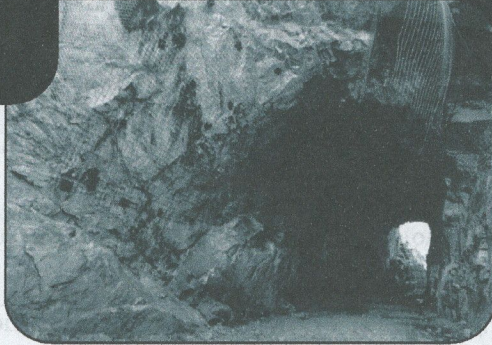
Interior of Needles Eye Tunnel, June 29, 2002. No rocks have fallen on the tunnel floor. Rockbolting on interior is performing as designed. Four inch mesh was bolted between rockbolts.
