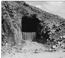
Needle's Eye Tunnel, East Portal
