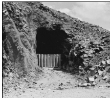
Needle's Eye Tunnel, East Portal
