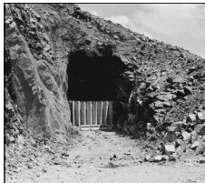
Needle's Eye Tunnel, East Portal
